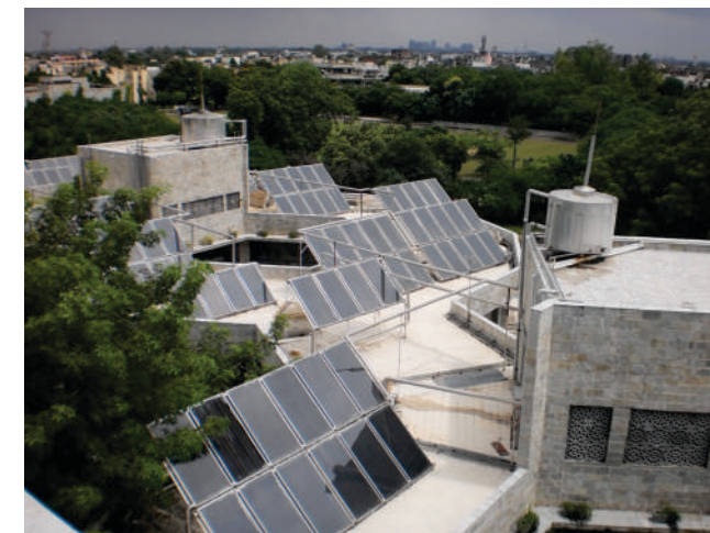
Collectors Installed in two in Inclined Plain South Facing to avoid shadows at Aurbindo Ashram New Delhi
