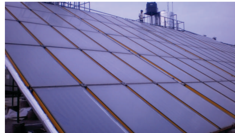
Solar Collector installed on South Facing Roof on structure supports inclined to get more effective Area
